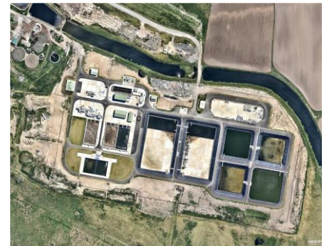
Nowra WwTP during upgrade
