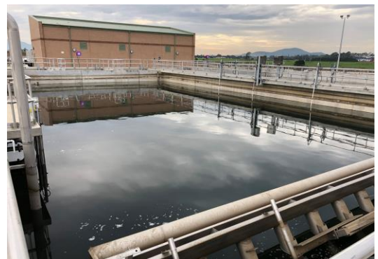
Bomaderry WwTP after completion
