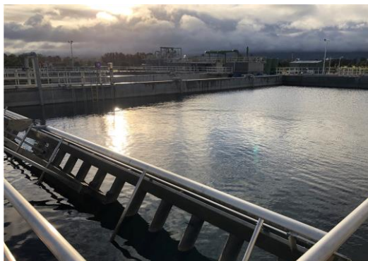
Nowra WwTP after completion
